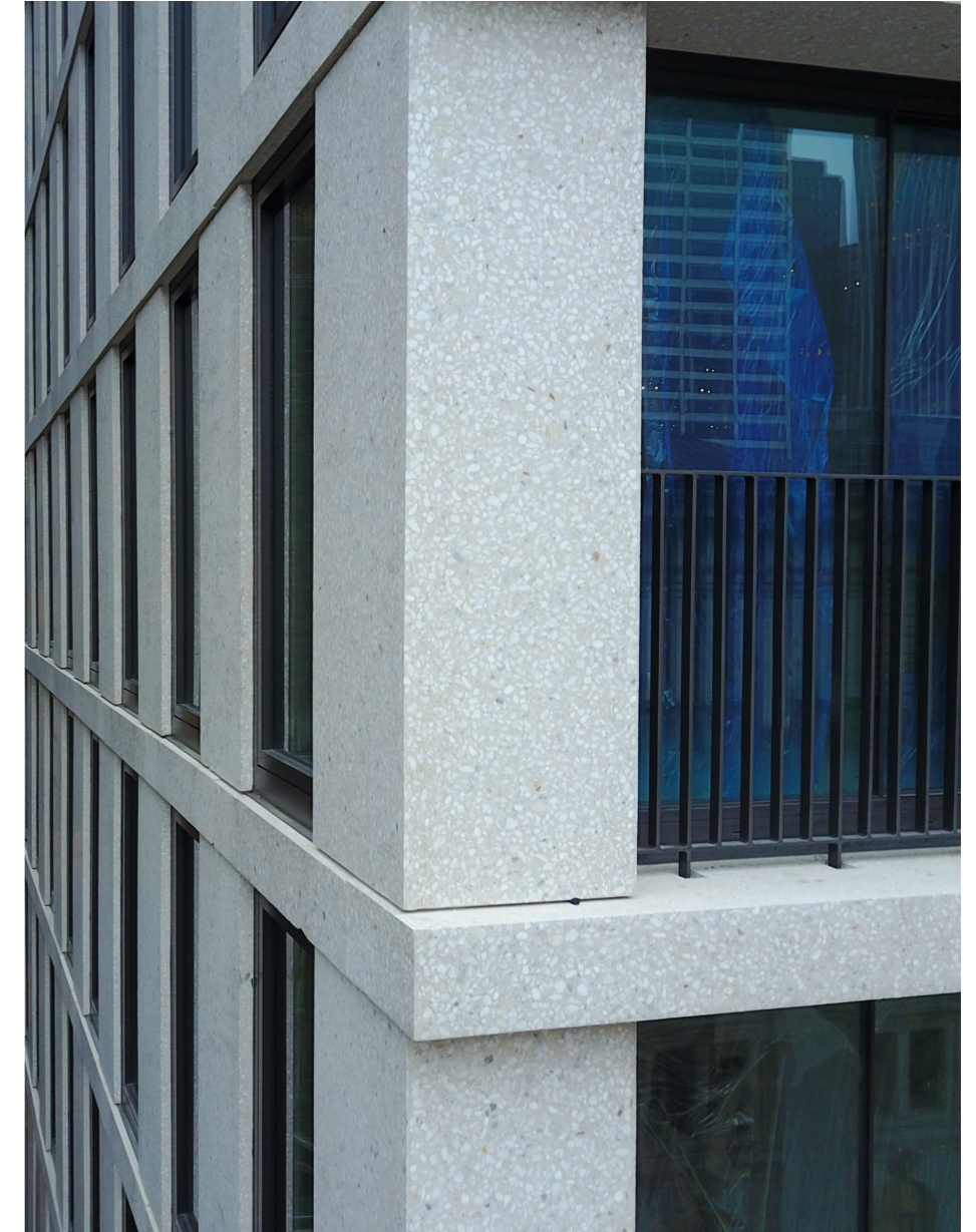
Precast Concrete Facade: The Bryant, New York
