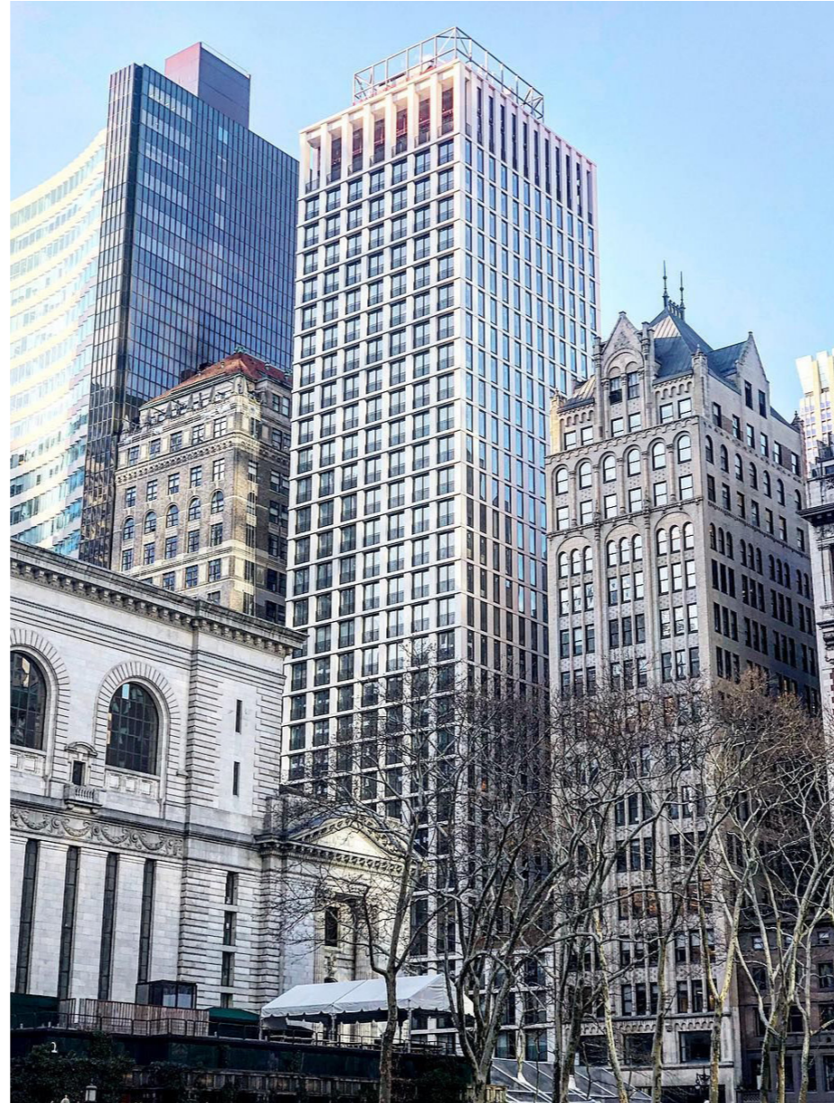
Precast Concrete Facade: The Bryant, New York
